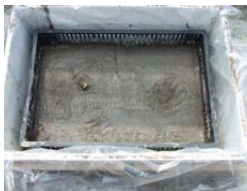
Casting a sink around a plastic crate
